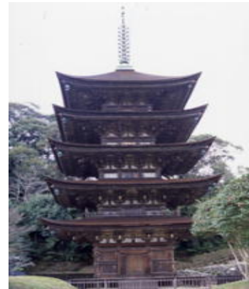
瑠璃光寺五重塔 Rurikoji, Five-Storeyed Pagoda
