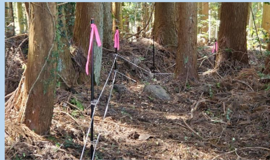
[イノシシ防護柵の点検・補修]
