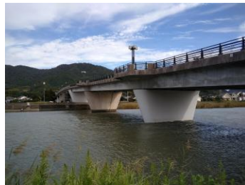
橋梁の耐震補強
